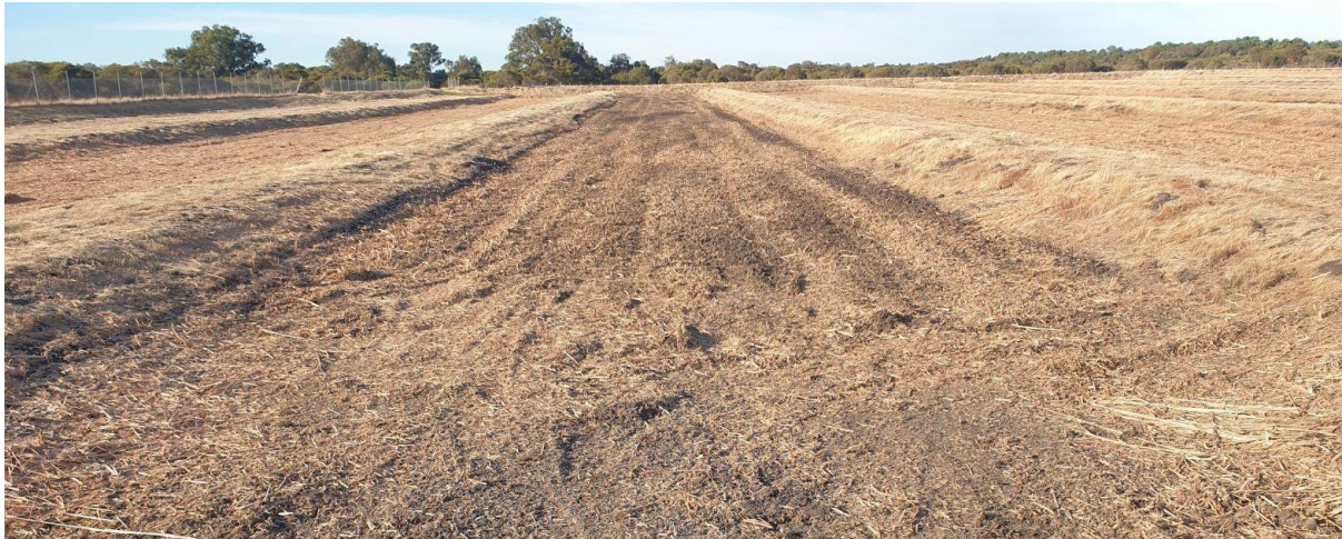
Figure 5 – Slashed & ripped Swale #2 (05/04/2024)
