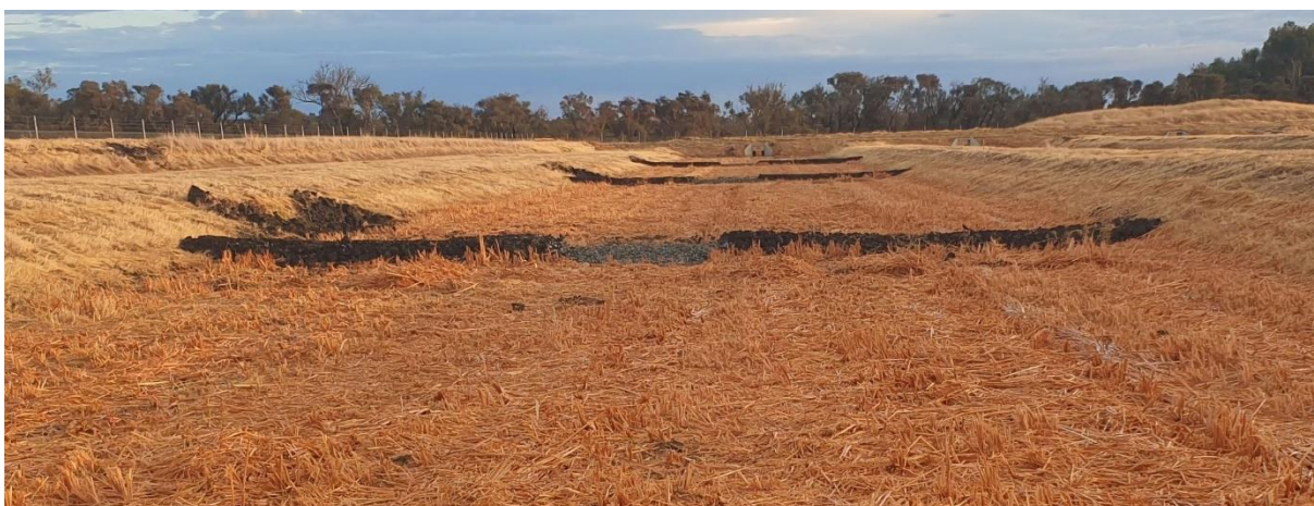
Figure 6 – Sloping Swale#6 – location of the three ‘riffles’ to create ponding (13/04/2024)
