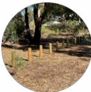
Bollards or large boulders for vehicle access control
