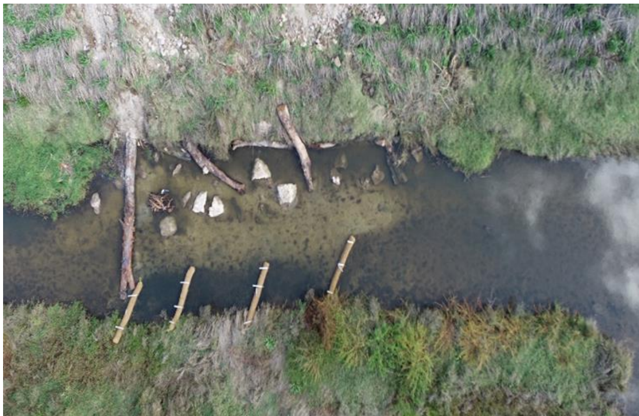
Installation of logs into the Lower Harvey River by the Harvey River Restoration Taskforce creates habitat for native fish
