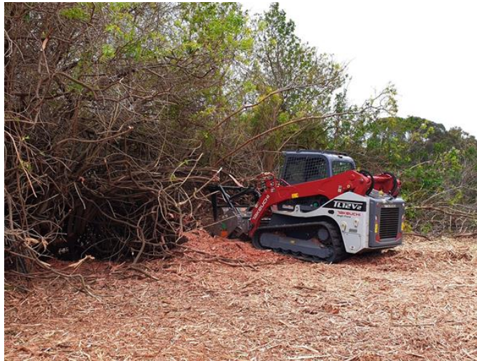
Removal of Brazilian Pepper thickets up to 4 metres high with heavy machinery near Lake Clifton
