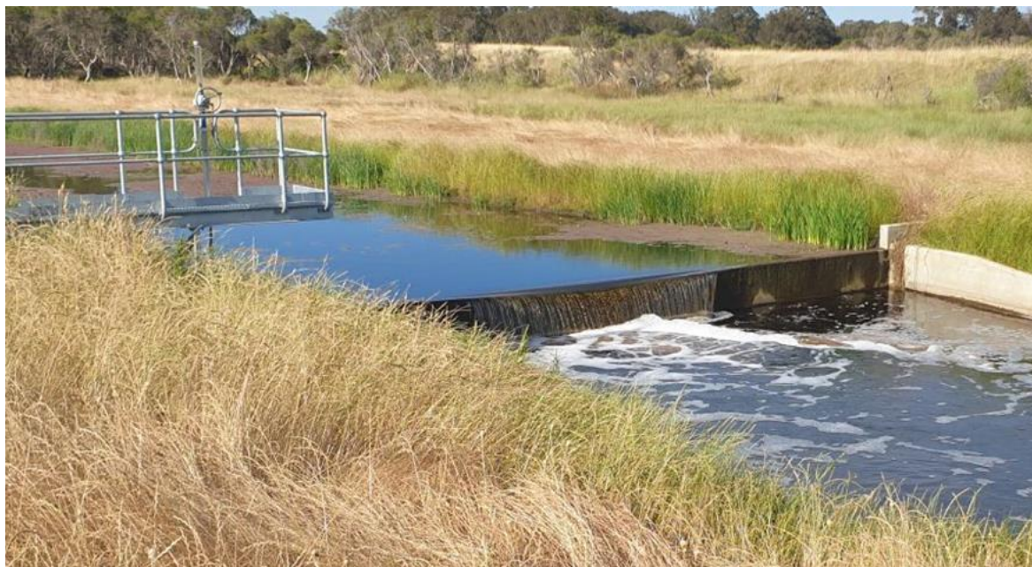
The weir constructed in the Peel Main Drain (shown above) diverts water into the treatment swales (below) designed to remove phosphorus from the drainage water
