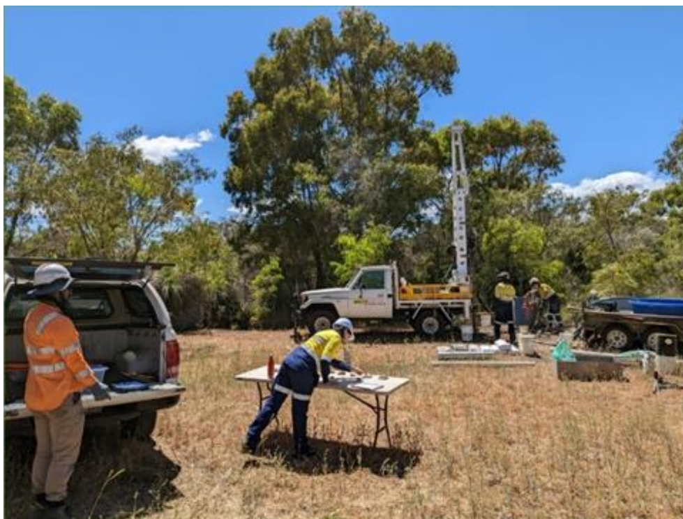
Installing groundwater bores at Lake Clifton as a precursor to hydrological investigations
