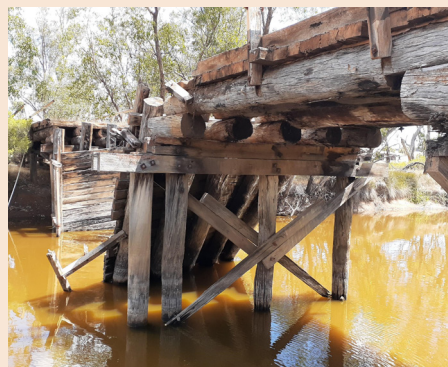
Old Pumphreys Bridge
