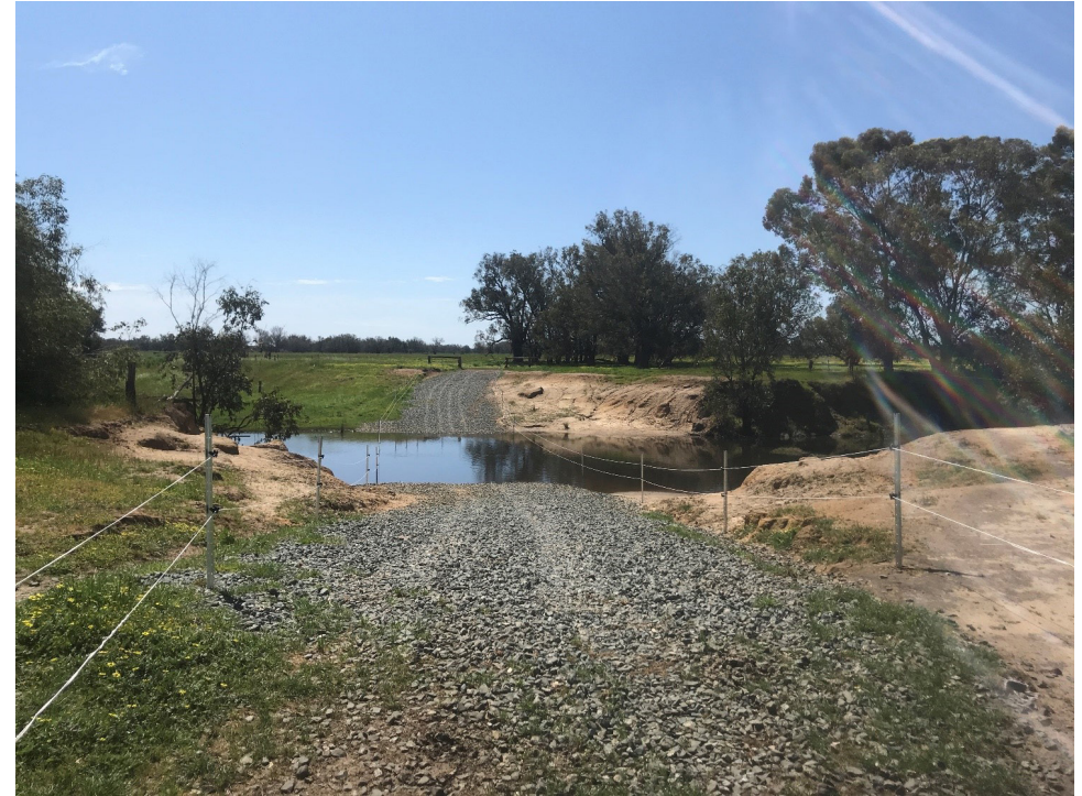
Figure 18: A cattle crossing restricting livestock from accessing the riparian zone.
