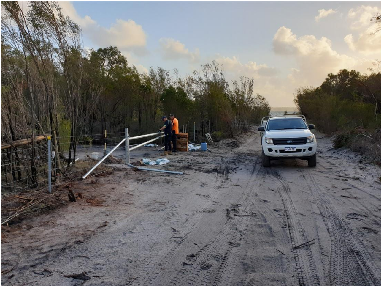
Contractors fit a gate to complete a fence line managing vehicle access into McLarty Nature Reserve near Harvey Estuary.
