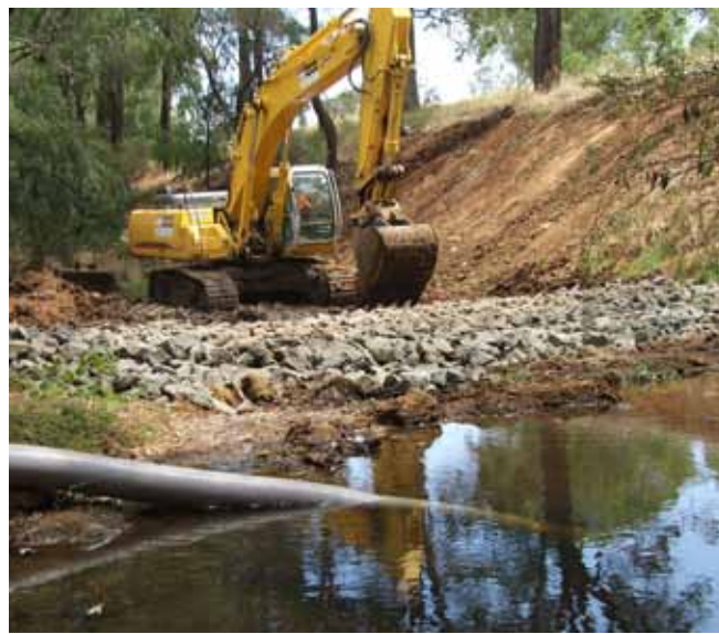
Example of Significant On-ground Works Managed by PHCC, Harvey River Riffle Installation, 2007.
