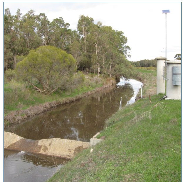
Coolup South Main Drain 613027 – May 2005
