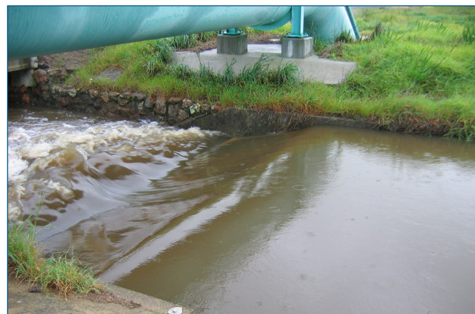
Samson North Drain at Somers Road – August 2005
