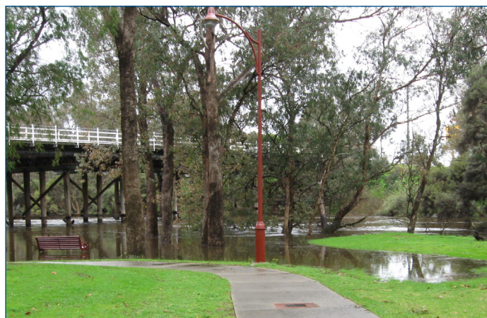
Flooding at Pinjarra, highest flow for the year – August 2009
