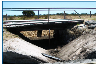
Before construction of the weir on Gull Road Drain (downstream view February 2005)
