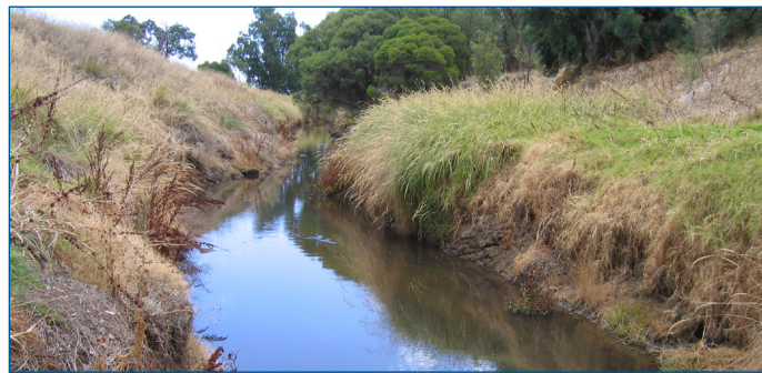
Upstream view of Waroona Drain at 6131335 – February 2008
