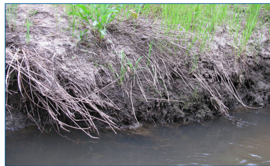
Erosion along Waroona Drain – October 2009
