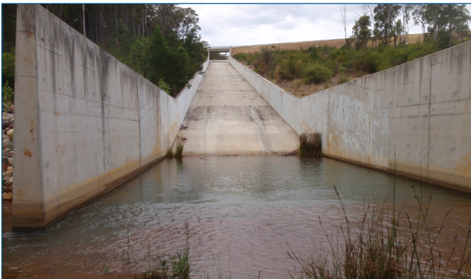
Above: Spillway from Waroona Dam
