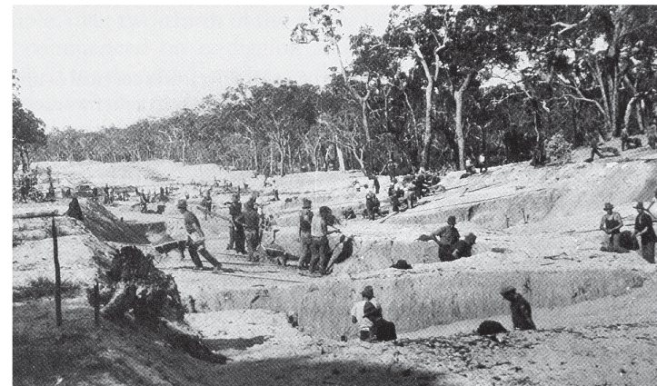
Construction of the Harvey River Diversion with axe, shovels and wheelbarrows during the depression in the early 1930s, courtesy of the Battye Library.
