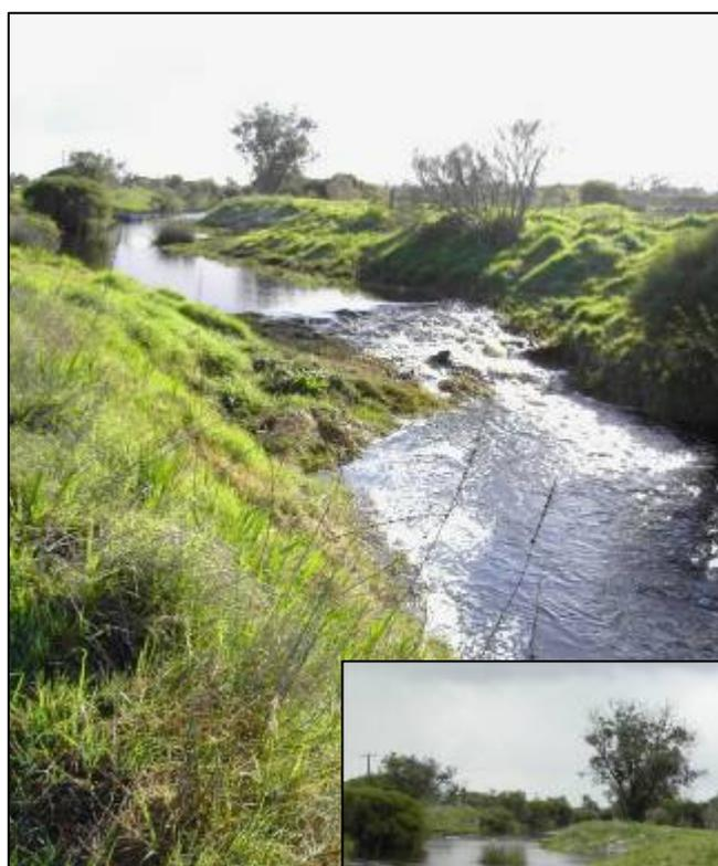
Figure 5: Artificial rock riffle on the Punrak Main Drain, Serpentine (winter base flow (left); high flow after winter storm (below))
